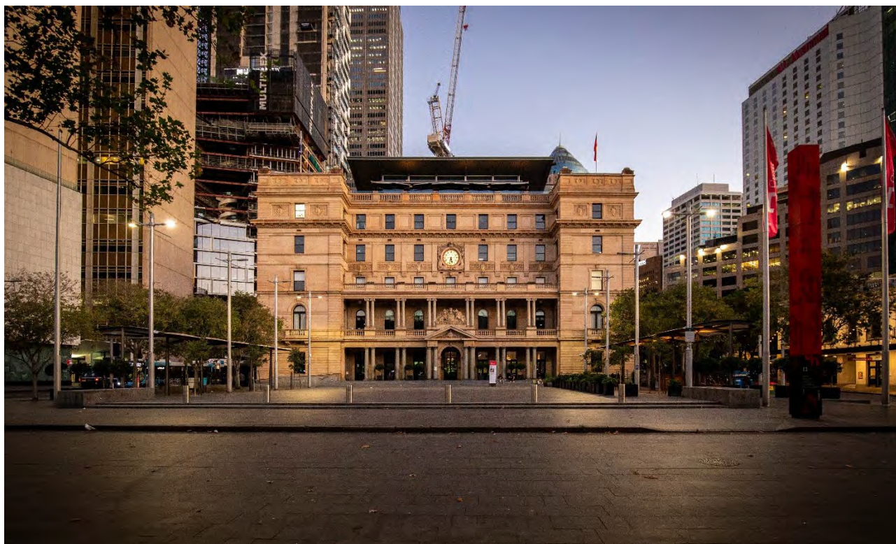
Figure 3. Customs House, Circular Quay – Photo by Katherine Griffiths / City of Sydney
